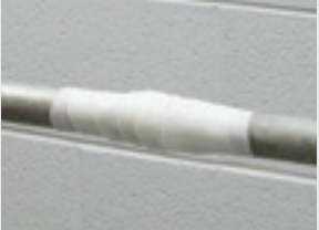
4. Finish off repair and let it cure.
